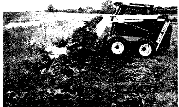
The digging up and filling in (as above) of a second set of drainage pipe lines last summer will help bring back some of the natural wetlands that once existed here.
