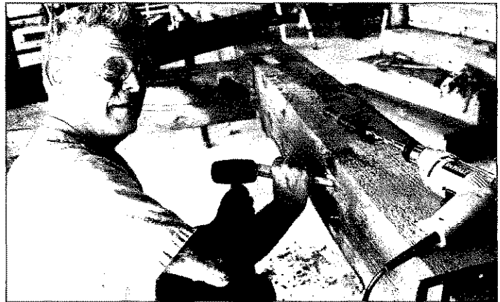
Mike Adolph chiseling a mortise joint.
